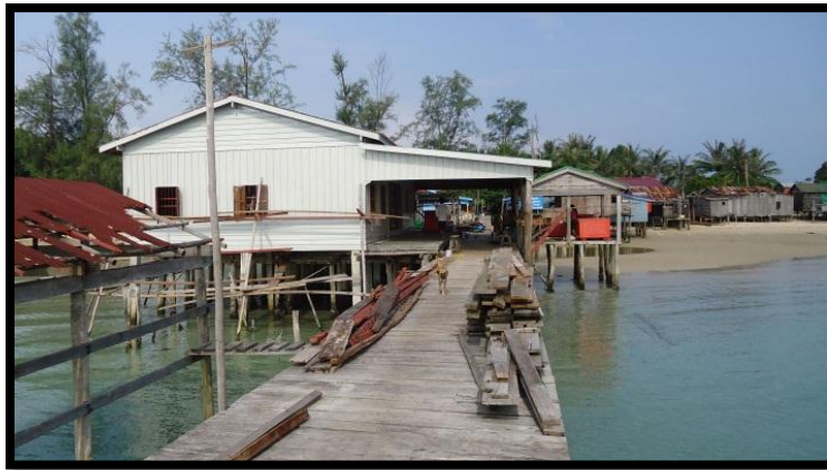
Photo 12 – Arrival at KRS CFI : main pier, June 2011
